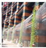
Mist generators have been installed to cool open spaces.
