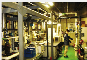
• Greywater plant (kitchen drainage reuse system)
